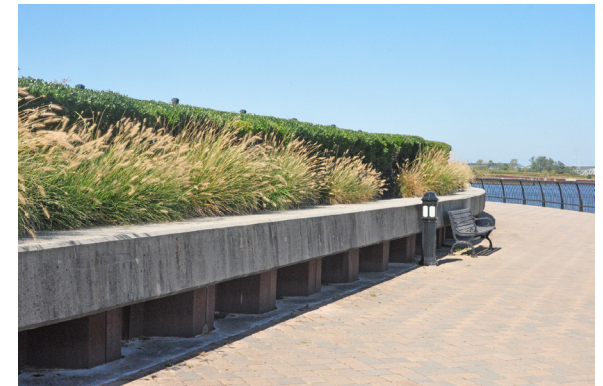
Floodwall constructed along Waterfront Walkway
