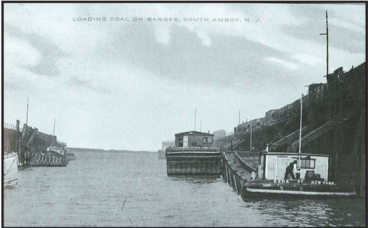
Photograph 5.19. Loading Coal on Barges. South Amboy, New Jersey. Circa 1900. (Source: Francy 1998).
