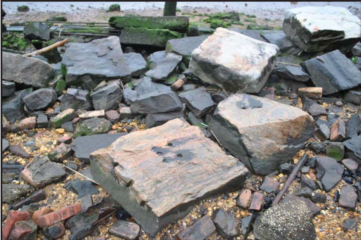
Photograph 7.13. Close-up view looking southeast showing Camden and Amboy Railroad stone sleepers used as backing for a wooden revetment probably constructed after the 1950 destruction of the explosives pier (Photographer: Patrick Harshbarger, May 2012) [HRI Neg. #11027/D1:14].
