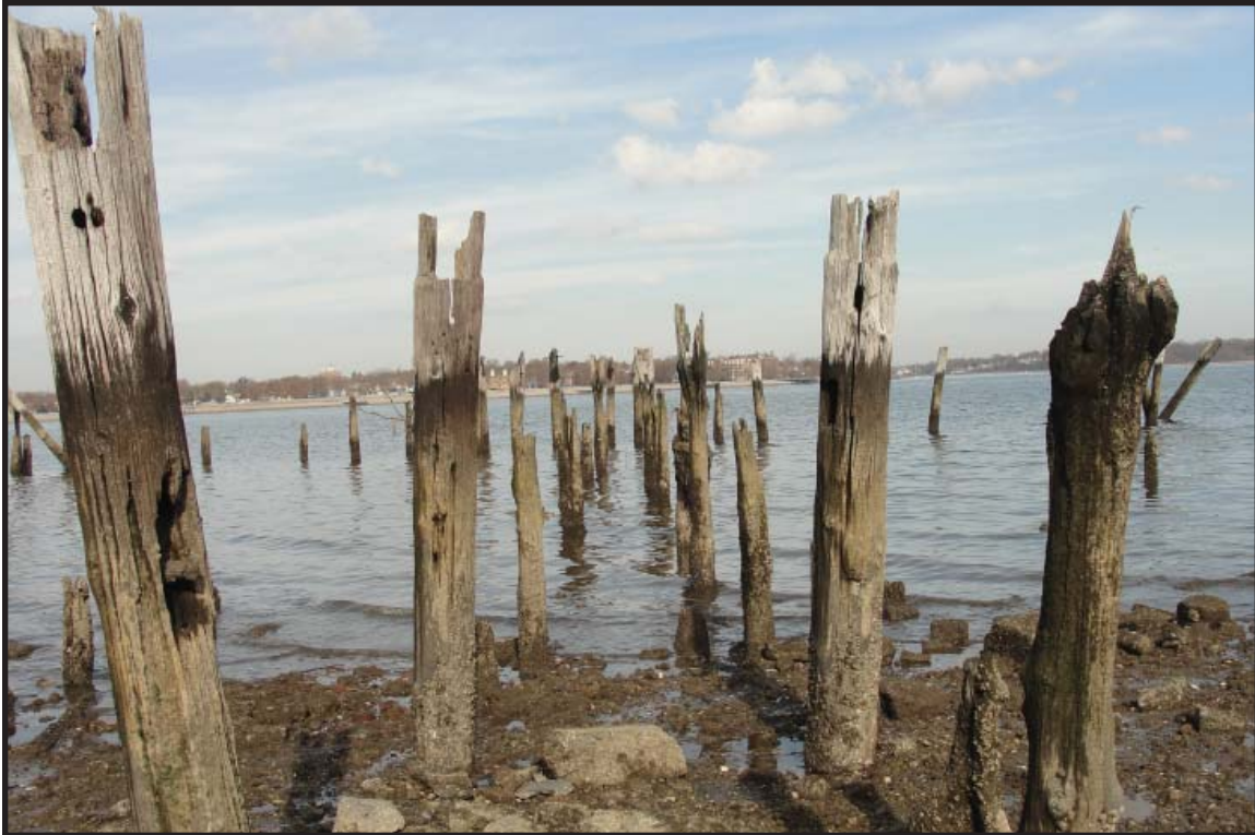
Photograph 7.5. View looking northeast toward Perth Amboy showing the timber supports for the pier which led to the c.1912 barge or “tie-up” racks built by the Pennsylvania Railroad to moor barges awaiting loading from the McMyler coal dumpers installed on the Lehigh pier to the south. The posts at right and left in the middle distance remain from the barge racks themselves (Photographer: Ian Burrow, October 2012) [HRI Neg. #11027/D5:DSC03634].
