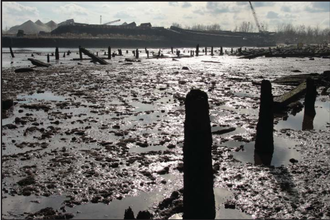
Photograph 7.9. View looking south showing the remains of the circa 1917-1950 explosives or powder pier, seen at low tide from the alignment of one of the 1870s Pennsylvania Railroad structures which supported additional sidings and the new freight house. The larger angled and vertical timbers are apparently part of the original wider explosives pier. This had been narrowed by 1950, possibly as a result of the 1923 explosion. The 1950 part of the pier is represented by the rather shorter posts beyond. Pier A (Westmoreland) is at rear, with several large barges washed onto it by Hurricane Sandy (Photographer: Ian Burrow, October 2012) [HRI Neg. #11027/D5:DSC03625].
