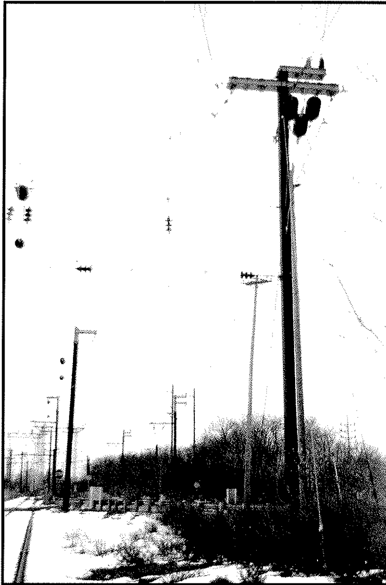
Plate 2. Catenary pole C8a. View facing northwest with poles C5 and C6 in the background. These originally single poles have had transmission structures added at the top. (Photographer: Ian Burrow, December 2002). [Hunter Research Inc. Negative 02081/1:22].
