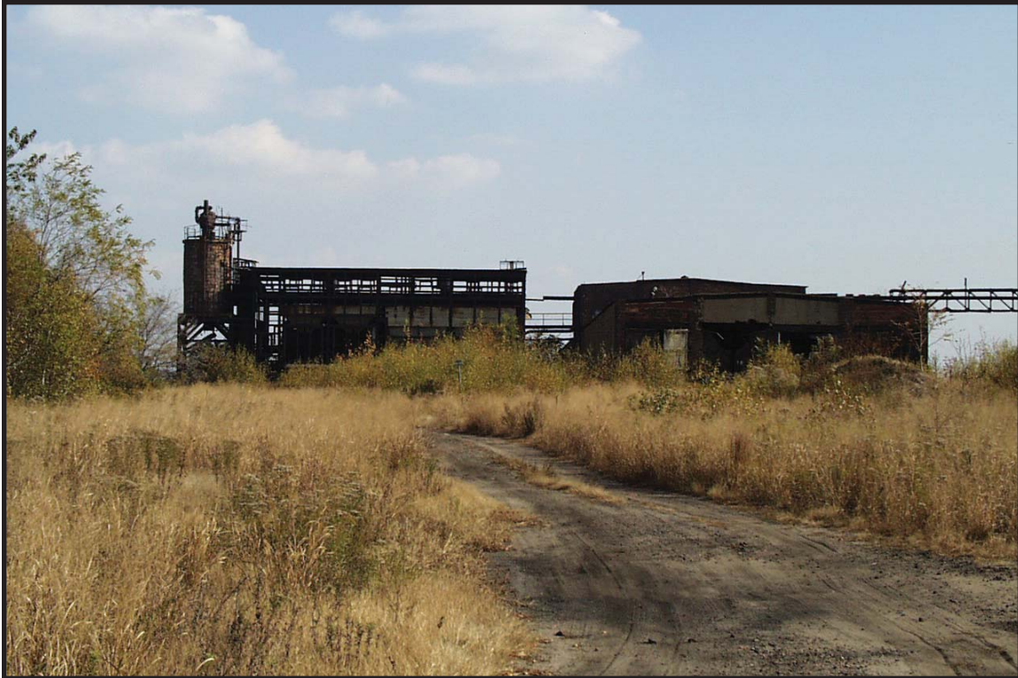
Photograph 6.2. General view looking east showing the relationship of the 1911 shed to the heating plant (Photographer: Ian Burrow, October 2001) [HRI Neg. #01005/D3:3].
