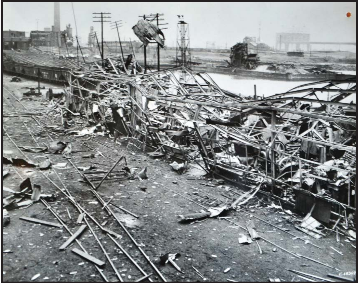
Photograph 5.35. Photograph, looking west, showing damage to the machine shop on the coal handling pier from the explosion of May 19, 1950 (Source: Pennsylvania Railroad Photographs Collection).
