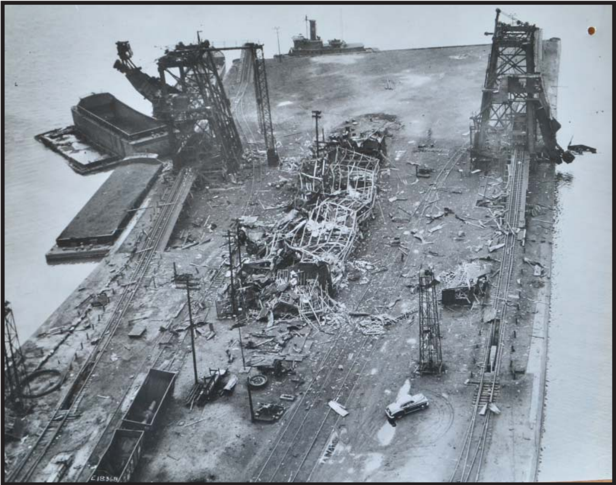
Photograph 5.34. Aerial view, looking down on the coal handling pier, showing damage from the explosion of May 19, 1950 (Source: Pennsylvania Railroad Photographs Collection).
