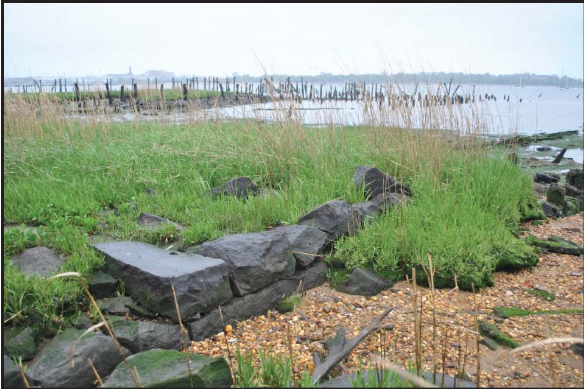
Photograph 7.7. View looking northeast showing the massive dressed stone masonry forming the onshore facing of the southeastern side of the 1870s Pennsylvania Railroad structure that supported additional sidings and a new freight house added to the existing Camden and Amboy Railroad passenger piers (Photographer: Patrick Harshbarger, May 2012) [HRI Neg. #11027/D1:19].
