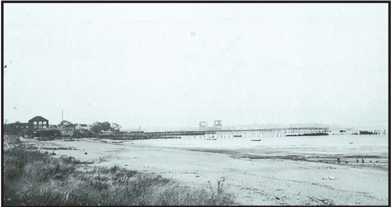
Photograph 5.22. Panoramic view of South Amboy shoreline with coal piers and dumpers in background, South Amboy, New Jersey. Circa 1920 (Source: Francy 1998).
