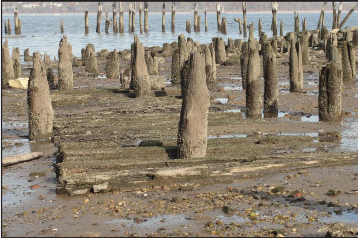
Photograph 7.3. View looking northeast showing the complex horizontal and vertical timbering in the area northwest of the barge rack pier. These support structures lie in the core area of the Camden and Amboy passenger terminal later used by the Pennsylvania Railroad, which also attached freight facilities to the southeast. Some of the timbers are probably of the pre-1871 Camden and Amboy Railroad era (Photographer: Ian Burrow, October 2012) [HRI Neg. #11027/D5:DSC03640].
