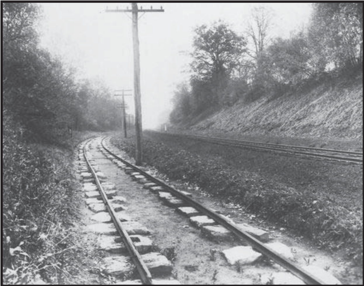
Photograph 5.6. Camden and Amboy Railroad track on stone sleepers near Jamesburg, New Jersey. Circa 1890 (Source: Smithsonian Institution Photograph Collections [Neg. # 21243-B]).
