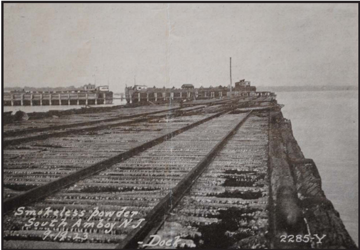
Photograph 5.28. Munitions pier at the Pennsylvania Railroad's South Amboy ferry terminal. 1923. View is looking northeast with the coal barge tie-up pilings in the background (Source: Dunn 1923).
