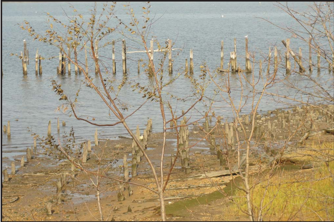
Photograph 7.1. View looking northeast from the shooting range mound showing the complex horizontal and vertical timbering in the area northwest of the barge rack pier (Photographer: Ian Burrow, October 2012) [HRI Neg. #11027/D5:DSC03653].
