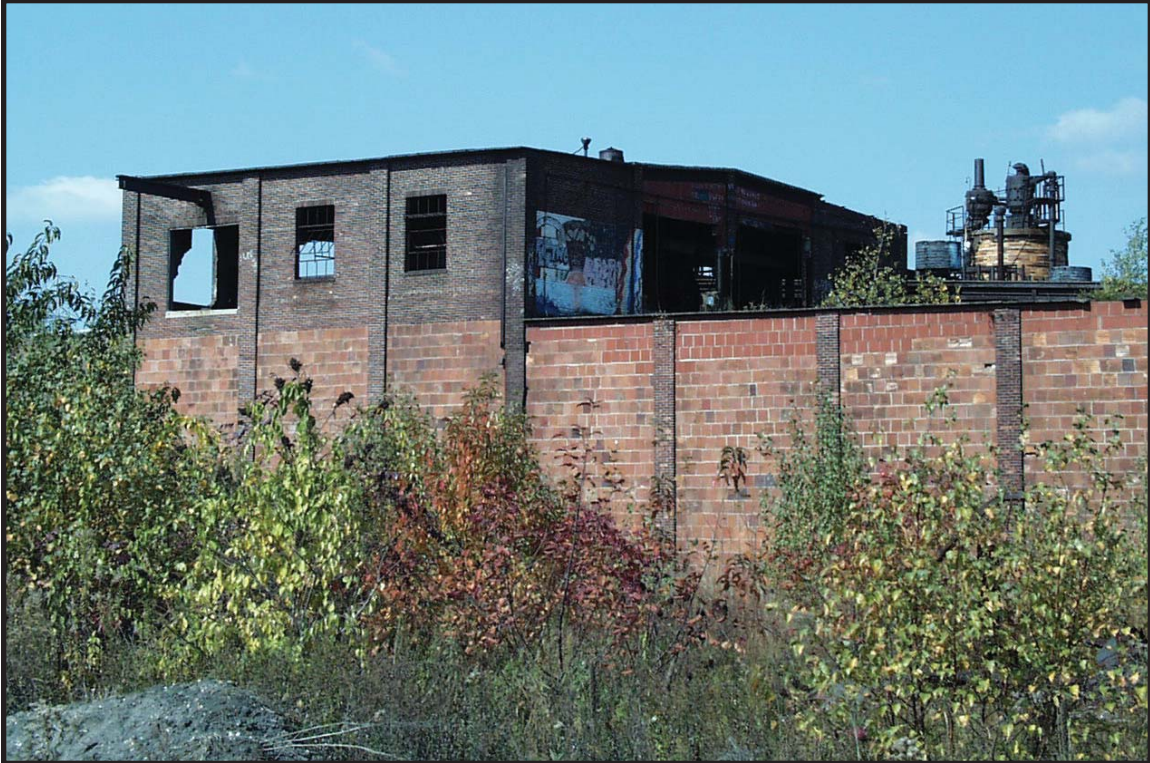
Photograph 6.3. View looking northwest showing detail of the superstructure of the 1911 shed (Photographer: Ian Burrow, October 2001) [HRI Neg. #01005/D3:14].
