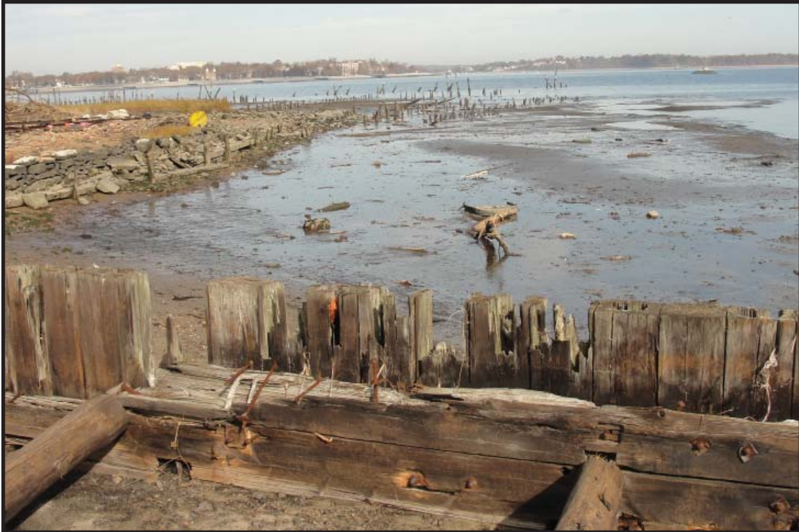
Photograph 7.11. General view looking east showing the site of the 19th-century Camden and Amboy Railroad and Pennsylvania Railroad piers and terminals. The timbering in the foreground is Pennsylvania Railroad-era bulkheading, possibly from the early 20th-century and associated with modifications related to the construction of the explosives or powder pier in 1917-18, fragmentary posts of which remain in the middle of the view (Photographer: Ian Burrow, October 2012) [HRI Neg. #11027/D5:DSC03613].
