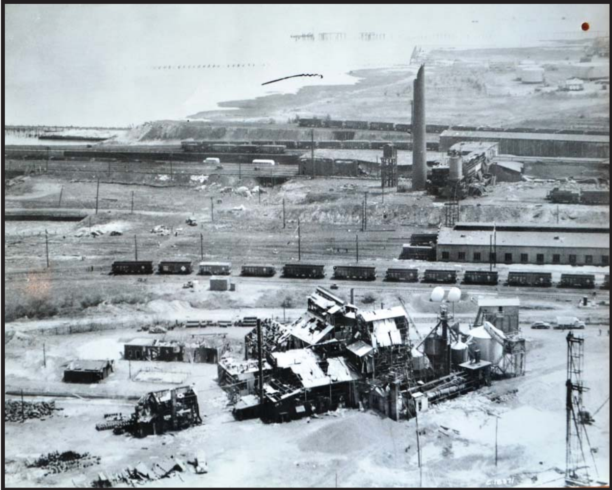
Photograph 5.36. Aerial view of the South Amboy ferry terminal, looking south, showing damage from the explosion of May 19, 1950 (Source: Pennsylvania Railroad Photographs Collection).
