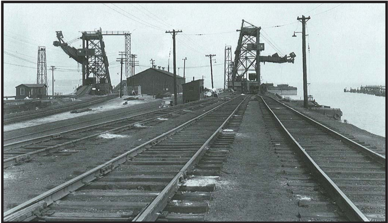
Photograph 5.41. View looking east at coal handling pier and dumpers. Circa 1953 (Source: Francy 1998).
