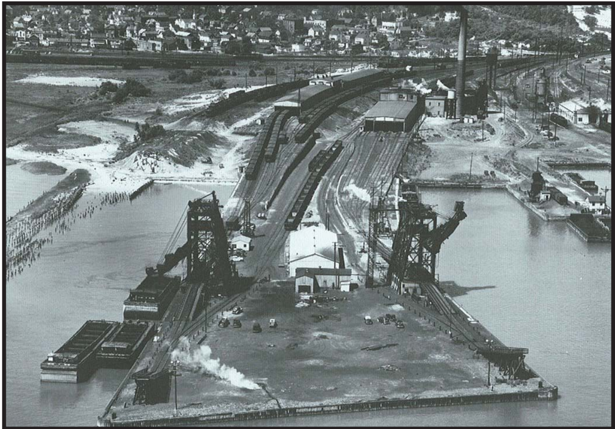
Photograph 5.40. Aerial view, looking west at coal handling pier. Circa 1953 (Source: Francy 1998).
