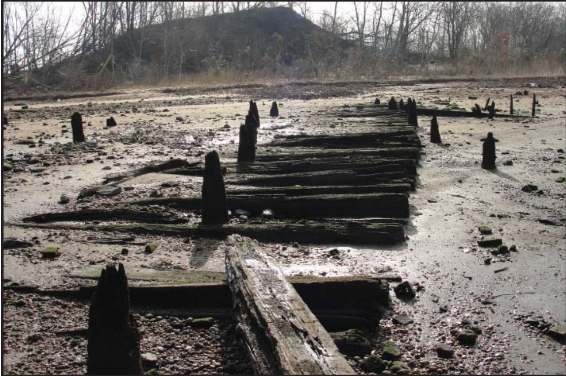
Photograph 7.4. View looking southwest at 180° from view in Photograph 7.3 showing mostly horizontal timbers probably placed by the Pennsylvania Railroad in the 1870s to form the northwest side of the expanded pier facilities. The large mound is a protective structure behind the targets of the police shooting range, which lies on the other side (Photographer: Ian Burrow, October 2012) [HRI Neg. #11027/D5:DSC03639].
