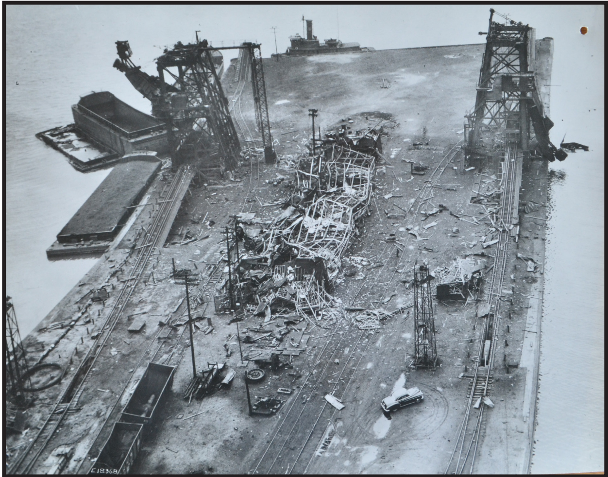
Figure 12. Aerial view looking down on the Lehigh Pier, showing damage from the explosion of May 19, 1950 (Source: Pennsylvania Railroad Photographs Collection).
