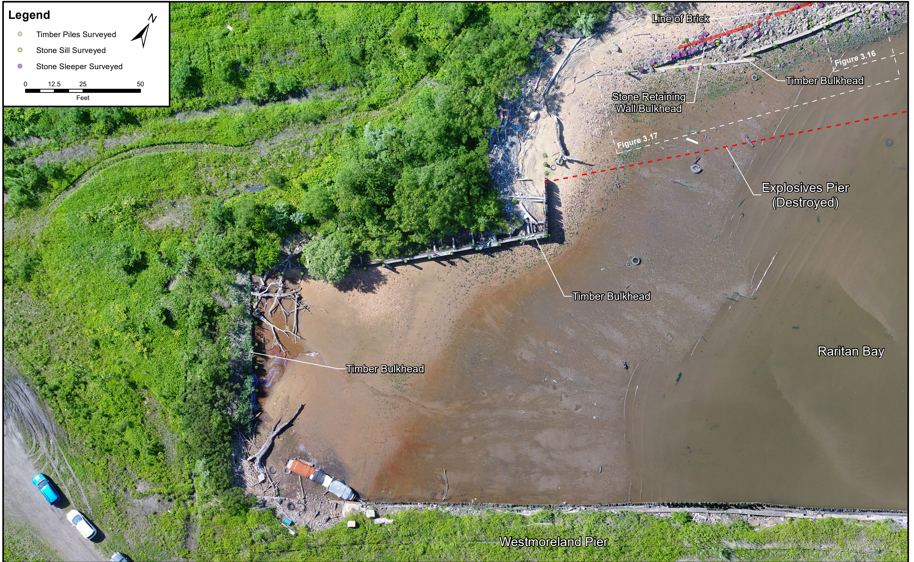
Figure 3.18. Aerial Photomosaic Plan View of the Inshore End of the Explosives Pier (Destroyed) and Bulkhead.
