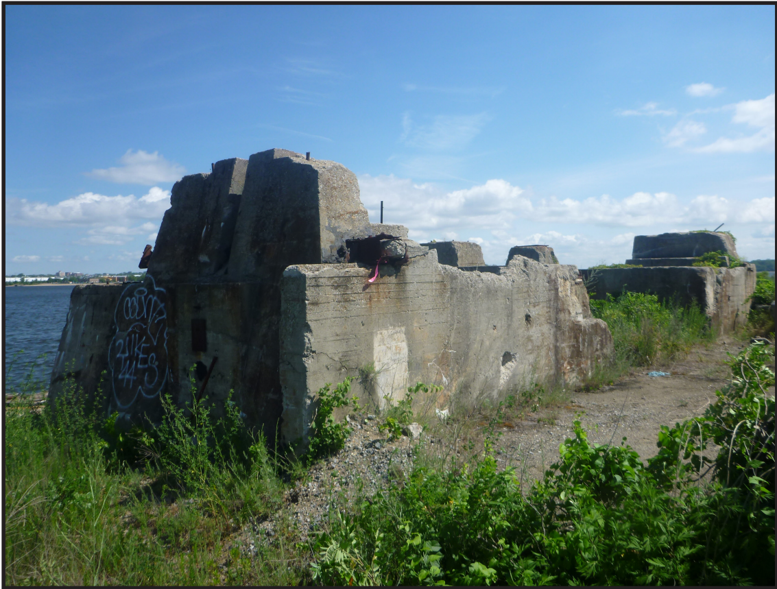
Photograph 3.46. Lehigh Pier: Dumper No. 1 foundations, view looking northeast (Photographer: Joshua Butchko, June 2020) [HRI Neg.# 19013/D8:036].
