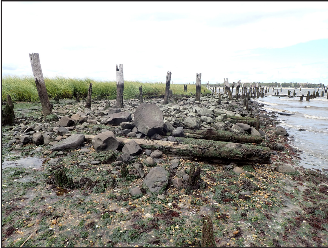
Photograph 3.16. View looking northeast showing the northeastern section of the bulkhead that defines the southeastern edge of the promontory. The double line of taller piles supported the catwalk connecting out to the barge rack, built circa 1920 (and may also have been part of the New Brunswick Pier, constructed in 1891). The short eroded vertical piles in the foreground suggest that this is a stub end of the bulkhead likely supporting one end of a trestle on which rail tracks were likely laid. These remains are interpreted as dating from the Camden and Amboy Railroad era, possibly from the early 1830s (Photographer: James Lee, September 2020) [HRI Neg.# 19013/D10:045].
