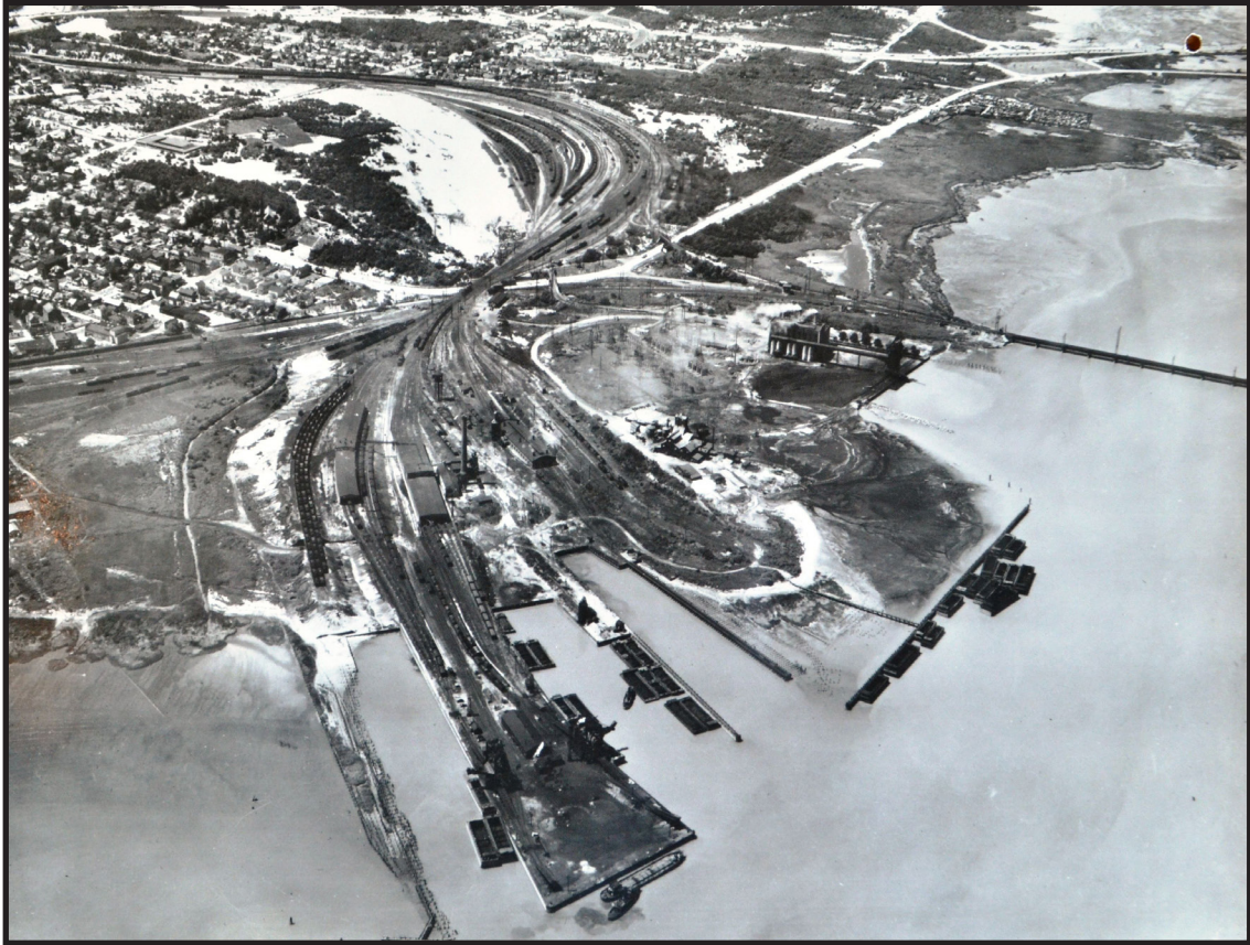
Photograph 4.6. Aerial view of the South Amboy Pennsylvania Railroad terminal, looking west, before the explosion of May 19, 1950. Source: Pennsylvania Railroad Photographs.
