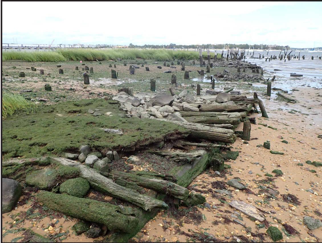
Photograph 3.14. View looking northeast showing the southwestern end of the bulkhead that defines the southeastern edge of the promontory. The vertical piles in the middle distance are part of Piling Structure A. The pile of stone just beyond the bulkhead remains in the foreground may represent the remains of a single crib box or pier base for a trestle. This bulkhead is interpreted as dating from the Camden and Amboy Railroad era, possibly from the early 1830s (Photographer: James Lee, September 2020) [HRI Neg.# 19013/D10:057].
