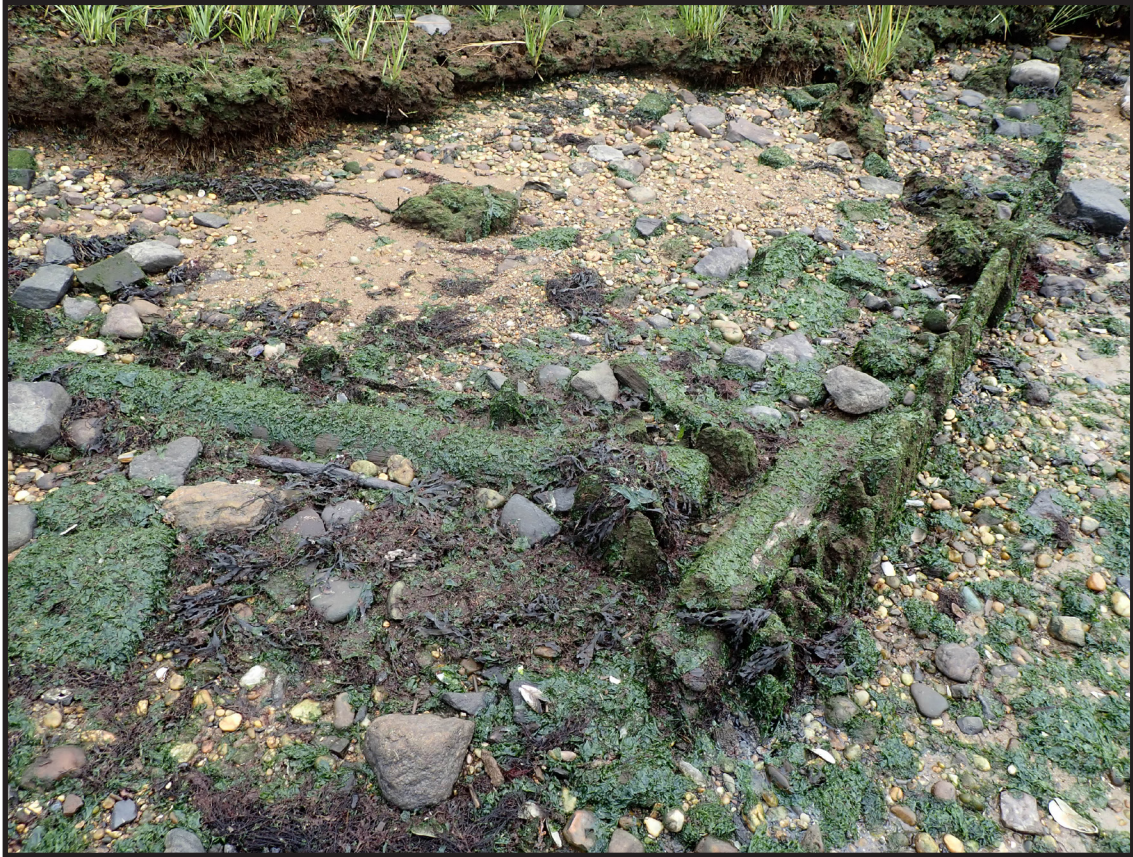
Photograph 3.13. View looking south along a section of timber bulkhead remains retaining the northwest side of the promontory. Note the timber sheeting at right along the outer edge of the bulkhead. These remains are separate from and define a narrower promontory than the remains shown in Photograph 3.12; on this basis they are thought to be older and may pre-date the Camden and Amboy Railroad era (Photographer: James Lee, September 2020) [HRI Neg.# 19013/D10:025].
