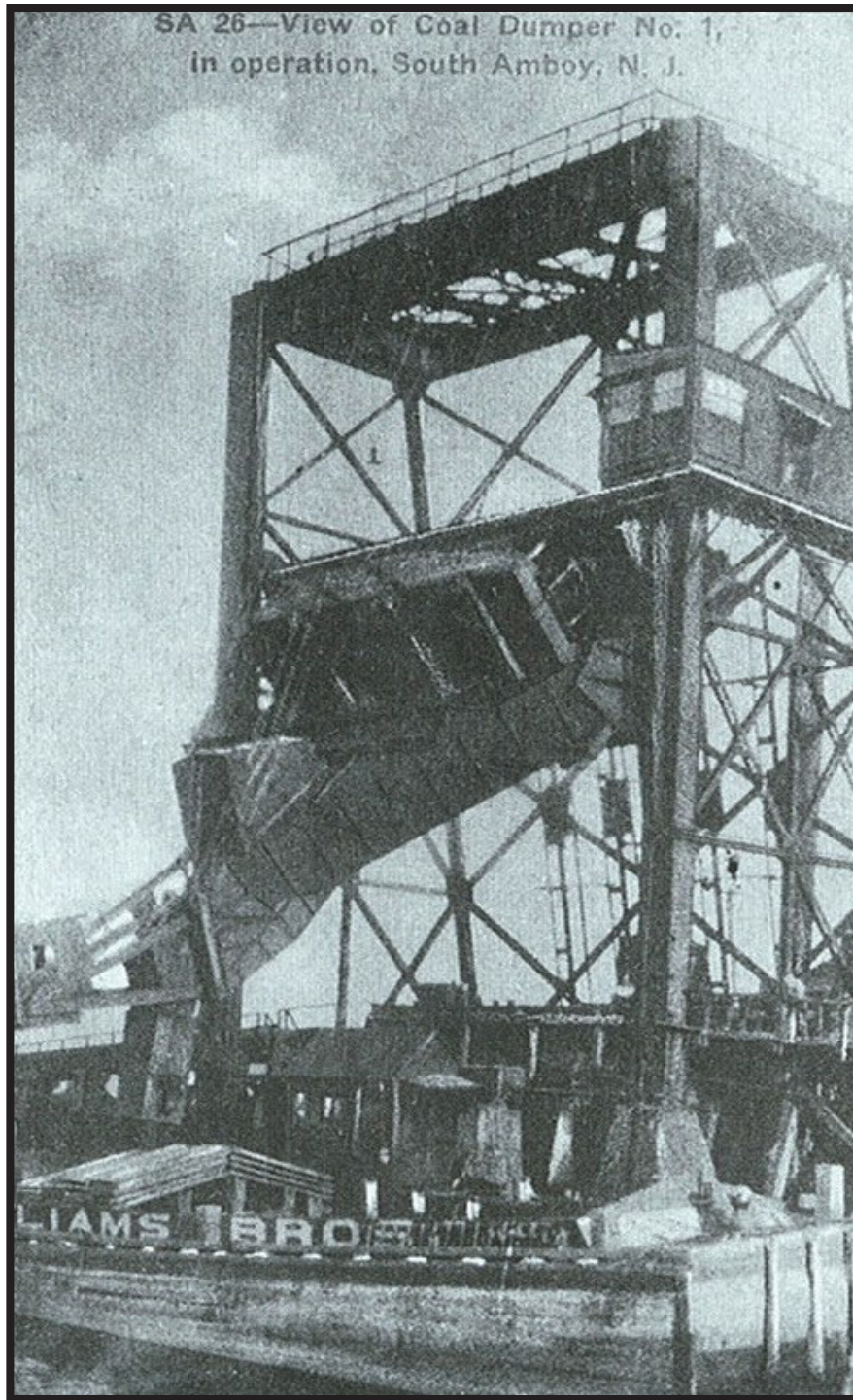
Figure 6. View of Coal Dumper No. 1 in operation on the Lehigh Pier, South Amboy, New Jersey. Circa 1920 (Source: Francy 1998).
