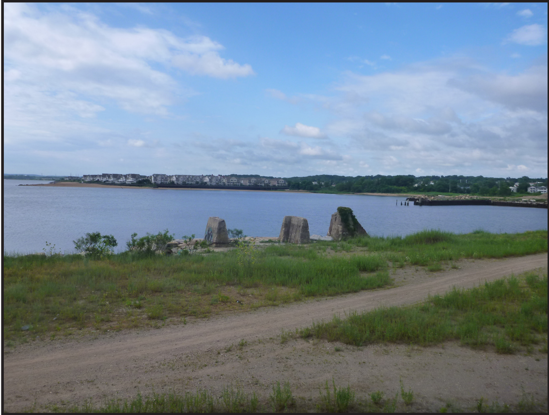
Photograph 3.47. Lehigh Pier: Dumper No. 2 foundations, view looking south (Photographer: Joshua Butchko, June 2020) [HRI Neg.# 19013/D8:007].
