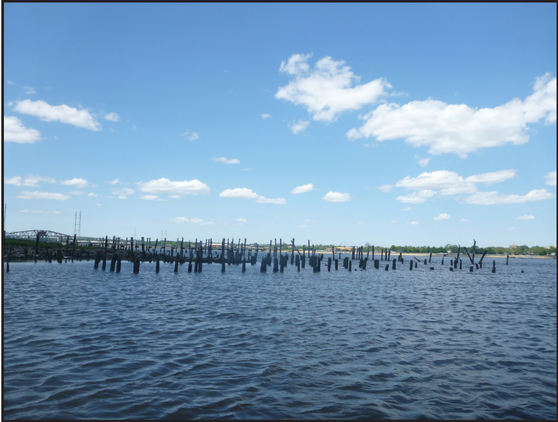
Photograph 3.19. View looking northwest towards Piling Structure B which lies just offshore and northeast of the promontory landform that supported the Camden and Amboy Railroad Ferry Terminal. These remains most likely date from the mid-19th century (Photographer: Joshua Butchko, June 2019) [HRI Neg.# 19013/D1:062].
