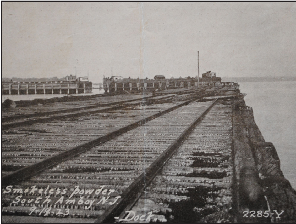
Photograph 4.5. The Pennsylvania Railroad freight pier, which was used as an explosives pier during and after World War I, following a fire in 1923. View is looking northeast with the barge rack in the background. Source: Dunn 1923.
