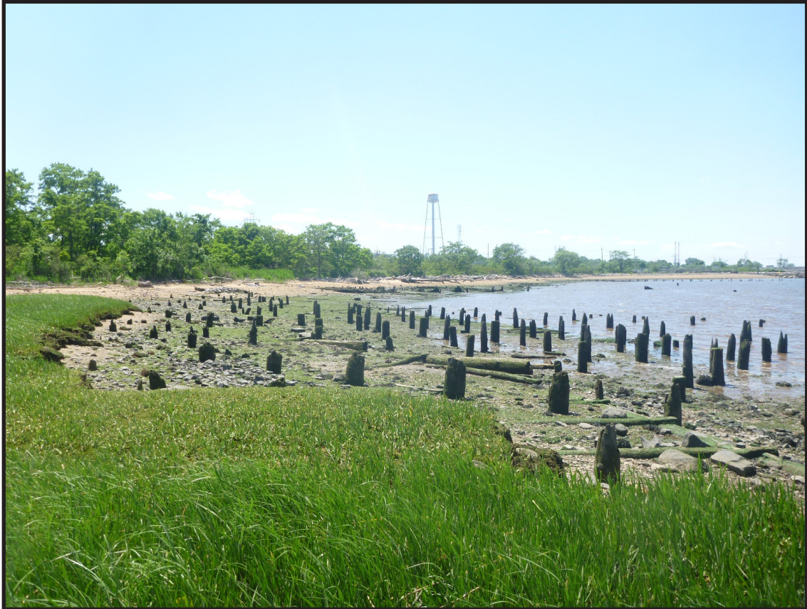
Photograph 3.11. View looking west along the Raritan Bay shoreline showing the pattern of timber piles forming Timber Piling Structure A which supported a major part of the deck for the Camden and Amboy Railroad/Pennsylvania Railroad terminal from the mid-19th century through circa 1890 (Photographer: Joshua Butchko, June 2019) [HRI Neg.# 19013/D1:082].
