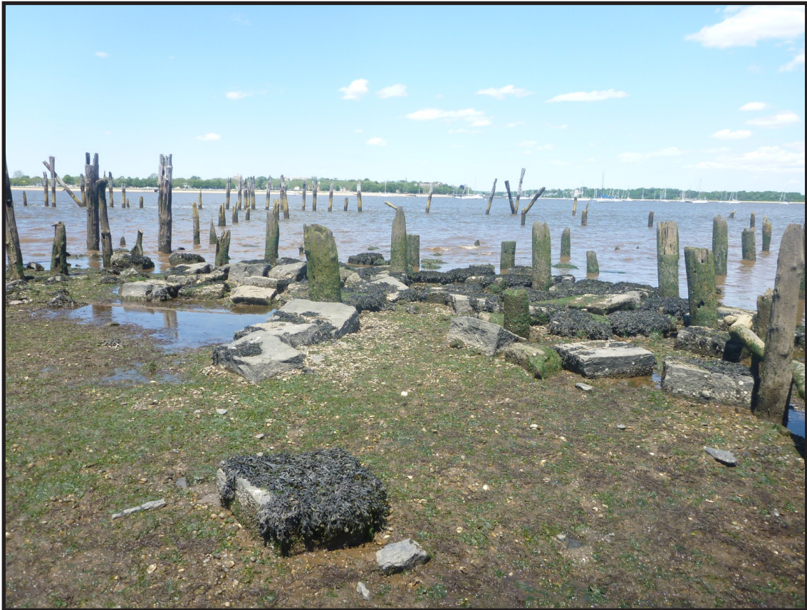
Photograph 3.20. View looking northeast showing the concentration of stone sleepers scattered amongst the piles of Piling Structure B just offshore and northeast of the promontory landform that supported the Camden and Amboy Railroad Ferry Terminal. Stone fragments such as these are thought to have been discarded on site in the course of later upgrades of the terminal facility (Photographer: Joshua Butchko, June 2019) [HRI Neg.# 19013/D1:080].
