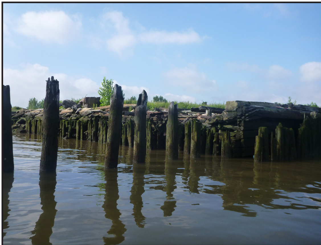
Photograph 3.39. Westmoreland Pier: view looking southwest at the northeast corner with the line of piles extending out to the left. This line of piles supported a walkway and a tie-up rack (Photographer: Joshua Butchko, August 2019) [HRI Neg.# 19013/D4:42].
