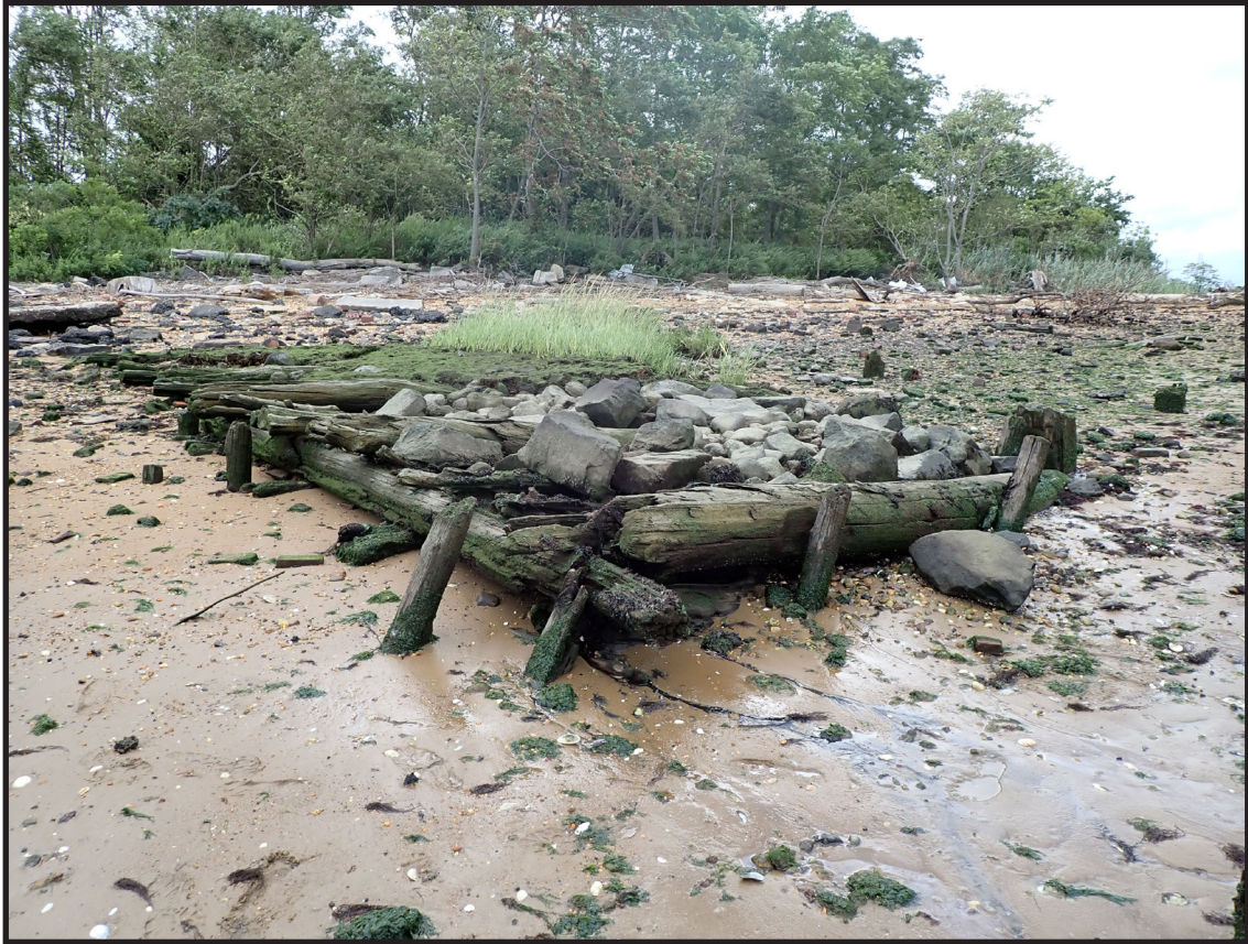
Photograph 3.15. View looking southwest showing the southwestern end of the bulkhead that defines the southeastern edge of the promontory. Note the vertical piles which suggest that this is a stub end of a section of bulkhead likely supporting one end of a trestle on which rail tracks were likely laid. These remains are interpreted as dating from the Camden and Amboy Railroad era, possibly from the early 1830s (Photographer: James Lee, September 2020) [HRI Neg.# 19013/D10:050].
