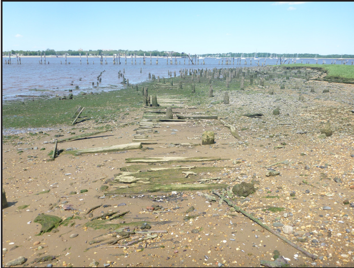
Photograph 3.8. View looking northeast along and down the alignment of the timber corduroy ramp thought to have been used to assist in launching and hauling vessels in and out of the bay. Note that timber piles from Piling Structure A have been driven through, and therefore post-date, the ramp. This ramp may date from the Camden and Amboy Railroad era or even from the 18th or early 19th centuries prior to the coming of the railroad (Photographer: Joshua Butchko, June 2019) [HRI Neg.# 19013/D1:093].
