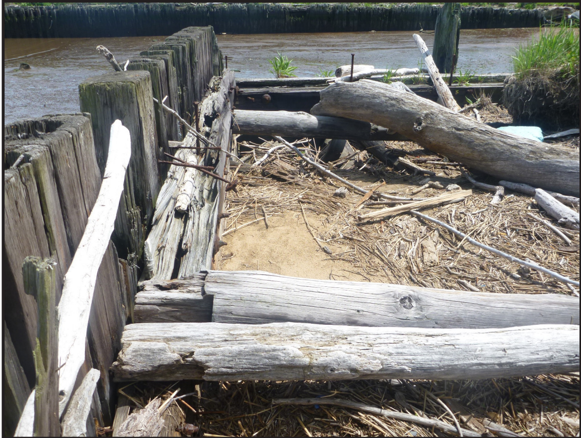
Photograph 3.32. View looking southwest showing the close-set vertical timber piles along the north-east face of the short segment of bulkhead from which the explosives pier, built in the mid-1920s, projected out into Raritan Bay (toward the camera). This section of bulkhead may originally date from the early 1870s and be contemporary with the Westmoreland and Lehigh piers (Photographer: Joshua Butchko, June 2019) [HRI Neg.# 19013/D1:218].
