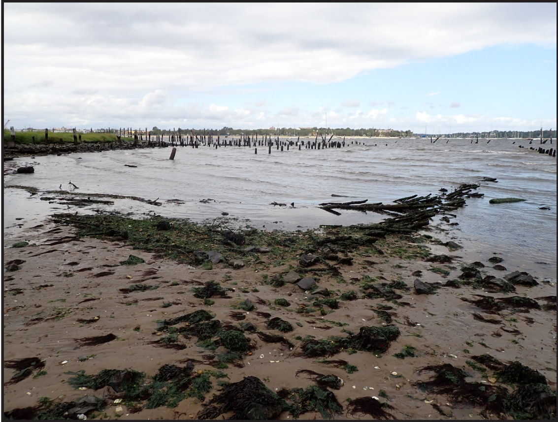
Photograph 3.24. View looking northeast showing the area of wood hurdles laid on the floor of the bay in the area of the railroad tracks leading to the Pennsylvania Railroad freight terminal. This feature may pre-date the Camden and Amboy Railroad era (Photographer: James Lee, September 2020) [HRI Neg.# 19013/D10:062].
