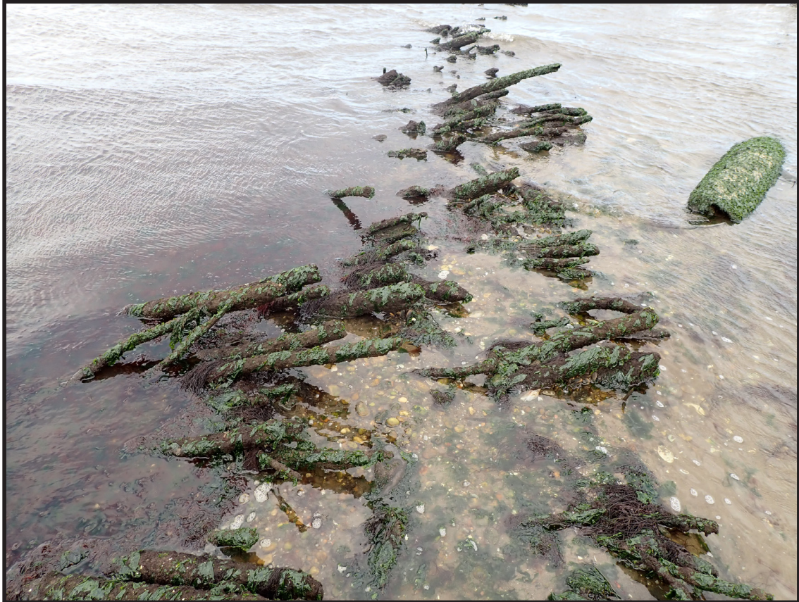
Photograph 3.25. Close-up view looking northeast showing the wood hurdles laid on the floor of the bay (Photographer: James Lee, September 2020) [HRI Neg.# 19013/D10:059].
