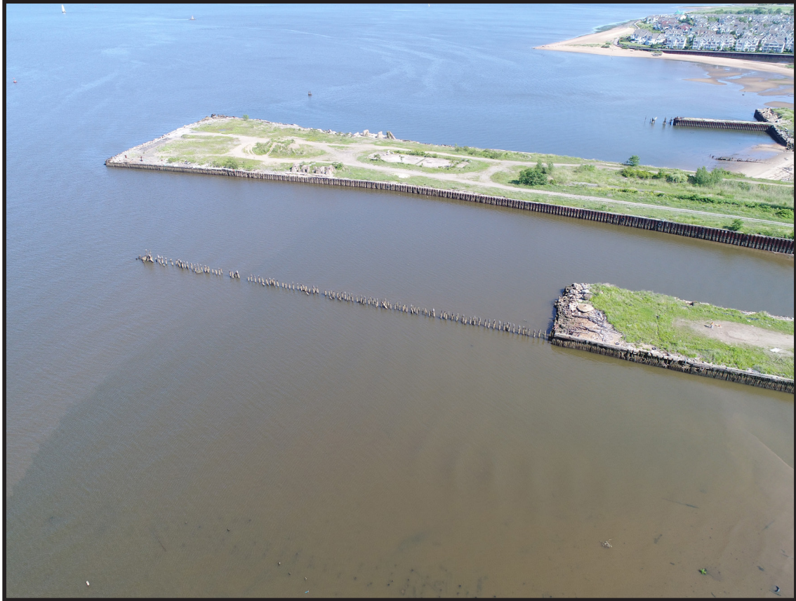
Photograph 3.43. Lehigh Pier: aerial view of the Lehigh Pier, center top of view, and the eastern end of the Westmoreland Pier and its tie-up rack piles, center of view (Photographer: Evan Mydlowski, June 2019 [HRI Neg.# 19013/DR1:608]).
