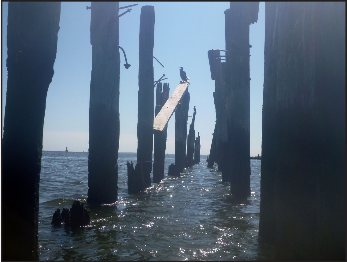
Photograph 3.2. View looking southeast along and between the two rows of piles that form the barge rack. Note the remnant transverse timbers hanging from some of the piles, the iron bolts with washers and nuts, and cormorants on the look-out for fish (Photographer: Joshua Butchko, August 2019) [HRI Neg.# 19013/D7:066].
