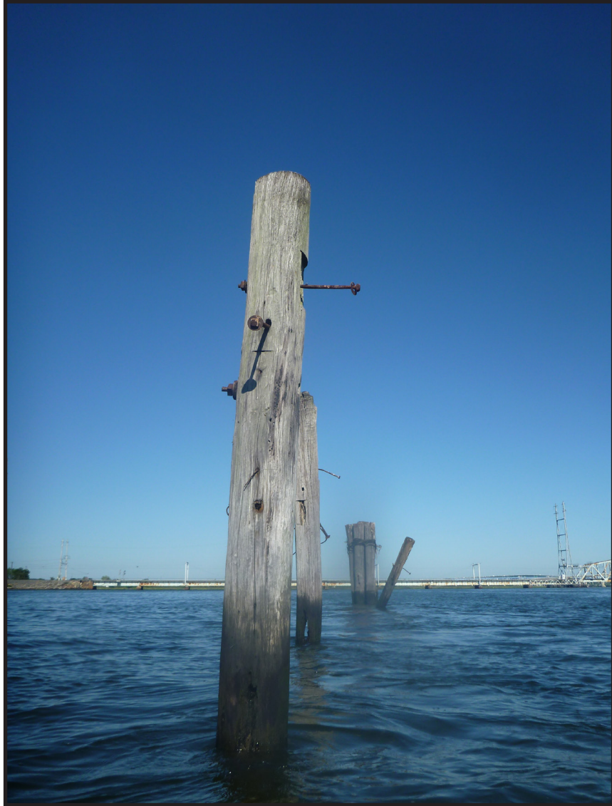
Photograph 3.5. View looking northwest showing a typical barge rack pile with iron hardware (bolts, nuts and washers) (Photographer: Joshua Butchko, August 2019) [HRI Neg.# 19013/D7:053].
