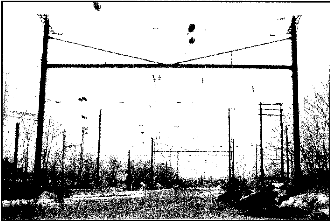
Plate 4. Portal Bridge Catenary C15a-b in foreground with C10a-b in background. View facing northwest (Photographer: Ian Burrow, December 2002). [Hunter Research Inc. Negative 02081/1:13].
