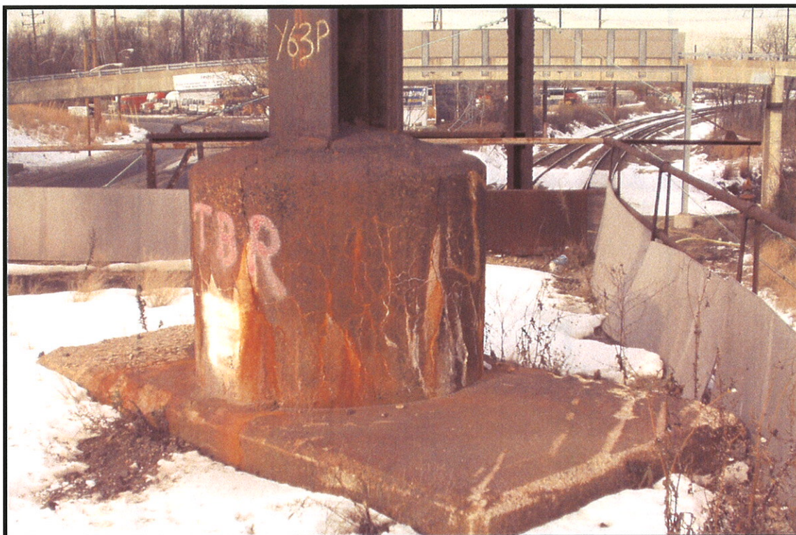
Plate 3. The base of Portal Bridge Catenary C10a from the southeast, showing concrete slab mat and concrete pedestal typical of Pennsylvania Railroad construction (Photographer: Ian Burrow, December 2002). [Hunter Research Inc. Negative 02081/D1:03].
