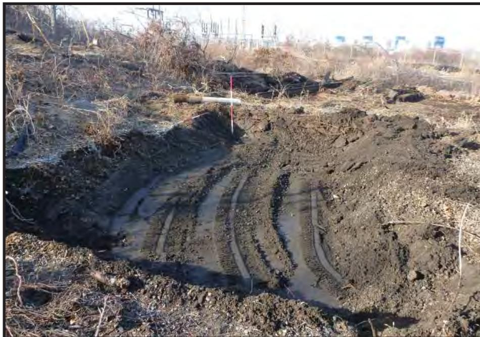
Photograph 5.8. View looking northwest showing Remedial Area 8 (AOC7-PHE 53) at the conclusion of excavation; no cultural features were observed; remediation occurred entirely within historic fill to a depth of between two and three feet; scale in feet (Photographer: Joshua Butchko, December 2016) [HRI Neg. #16008/D5:173].
