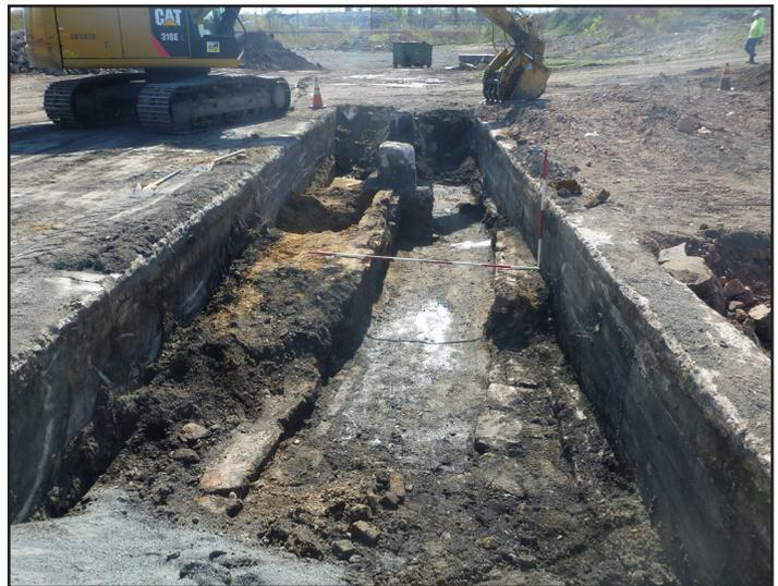
**Left:** The southern portion of the mid-19th-century turntable pit beneath the concrete floor of the engine house. **Right:** The mortared brick and stone foundation supporting the approach track leading into the mid-19th-century turntable. [Source: Hunter Research, Inc.].
