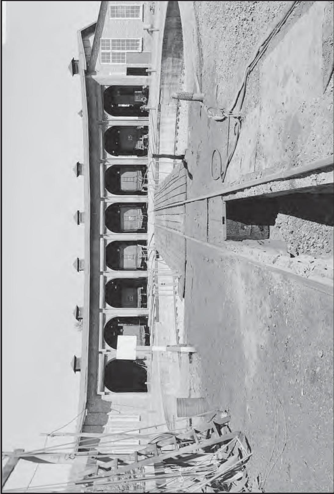
Photograph 3.49. Typical view of a turntable with ash pit beneath an approach track at the East Broad Top Railroad & Coal Company Roundhouse, Rockhill Furnace, Huntingdon County, Pennsylvania (Source: Boucher 1986) [HAER PA, 31-ROCFN, 1B--8]).
