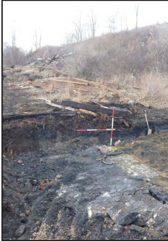
Photograph 5.20. View looking west-northwest showing the western end of Remedial Area 17 (PHE Area 1); the concrete floor and brick and stone foundation of the machine shop [Structure 43] are visible in the foreground; remediation in this area occurred within historic fill and contaminated natural sands to a depth of three feet; scales in feet (Photographer: Joshua Butchko, December 2016) [HRI Neg. #16008/D7:413].
