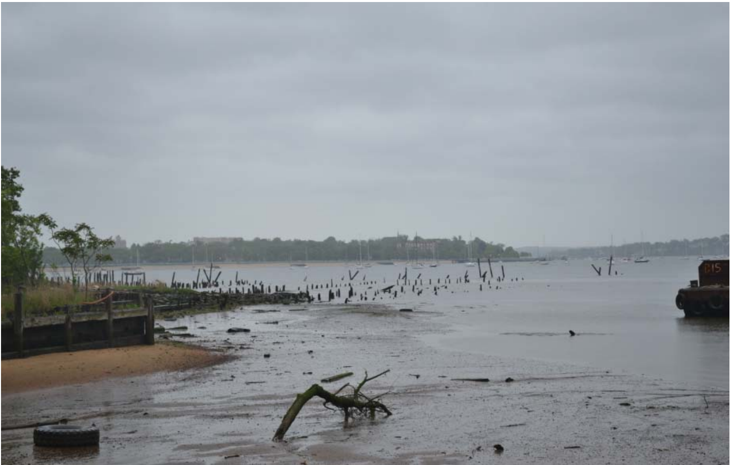
This 2012 photograph shows the north side of the project area looking toward Perth Amboy. The pilings mark the approximate location of the original Camden and Amboy Railroad T-wharf. [Source: Hunter Research, Inc.].
