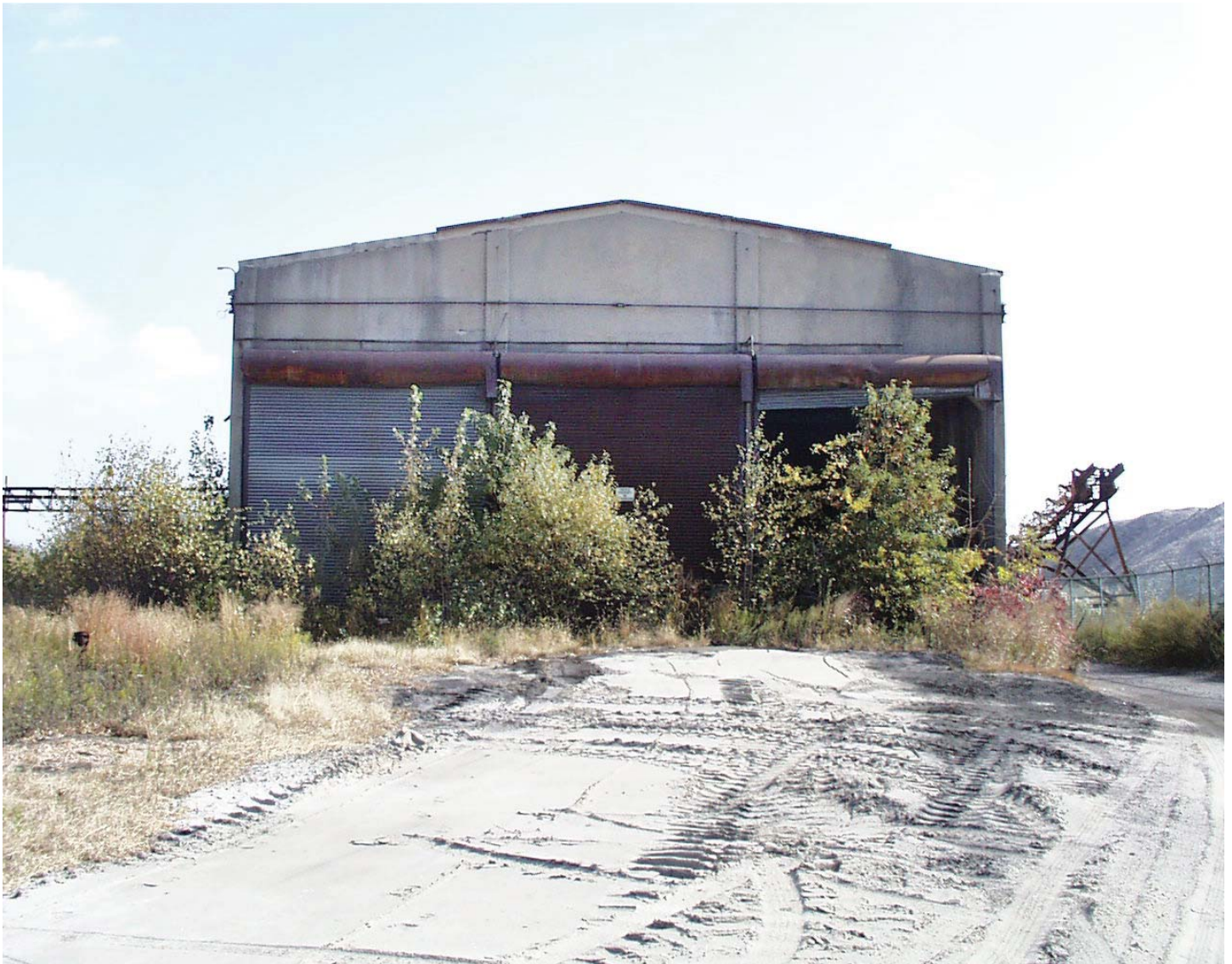
This 2001 photograph shows the western end of the 1916 coal thawing shed. It was torn down prior to 2012. [Source: Hunter Research, Inc.].
