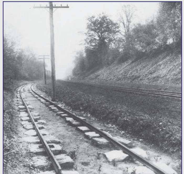
Camden and Amboy Railroad track on stone sleepers near Jamesburg, New Jersey. Circa 1890. [Source: Smithsonian Institution].
