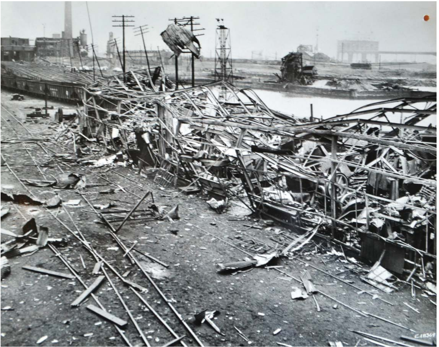
This photograph, looking west, shows the damage to the machine shop on the coal-dumper pier from the explosion of May 19, 1950. [Source: Pennsylvania Railroad Photographs Collection, Hagley Library and Archives].
