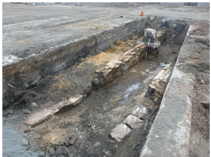
Left: View looking west showing the southern portion of the mid-19th-century turntable pit beneath the concrete floor of the engine house. Right: View looking southwest showing the mortared brick and stone foundation supporting the approach track leading into the mid-19th-century turntable. [Source: Hunter Research, Inc.]
