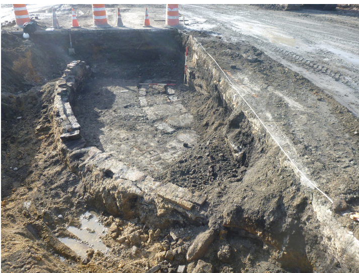
Left: View looking west showing the southern portion of the mid-19th-century turntable pit beneath the concrete floor of the engine house. Right: View looking southwest showing the mortared brick and stone foundation supporting the approach track leading into the mid-19th-century turntable. [Source: Hunter Research, Inc.]
