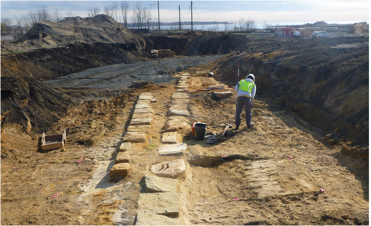
View looking east showing the junction of the two lines of stone sleepers. [Source: Hunter Research, Inc.]
